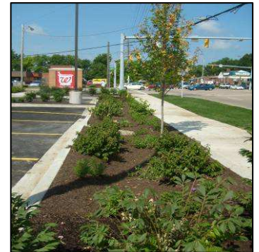
Open curb allows parking lot runoff into the bioswale to filter pollutants
