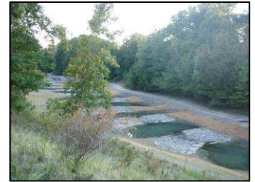
Wetland Retrofit - After
