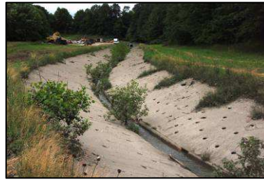
Detention Basin - Before
