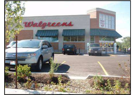
Open curb allows parking lot runoff into the bioswale to filter pollutants
